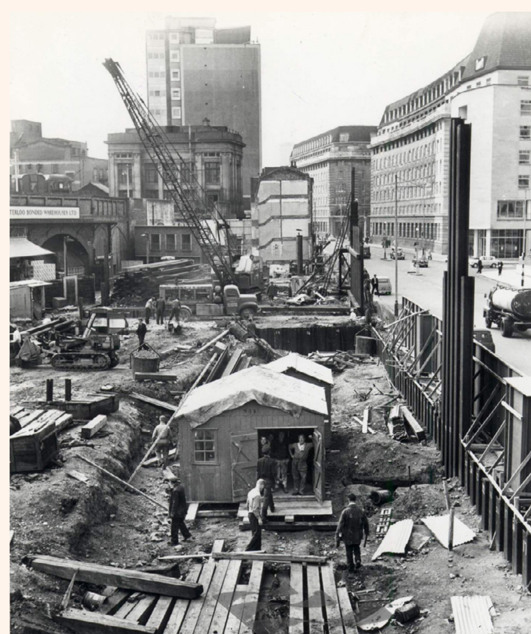
Elizabeth House was built.
